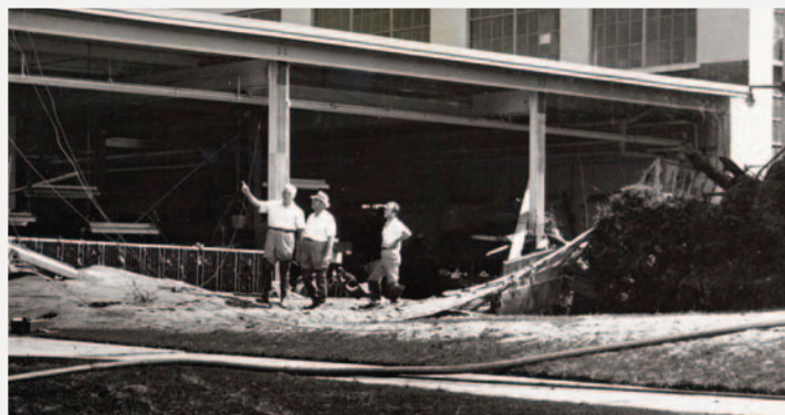
Mr. Frey, Mr. Hershey, and Mr. Goodkind surveying the damage to Hershey Metals after the 1955 flood.
